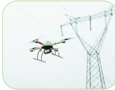
UAV-based inspection robot system (China)
