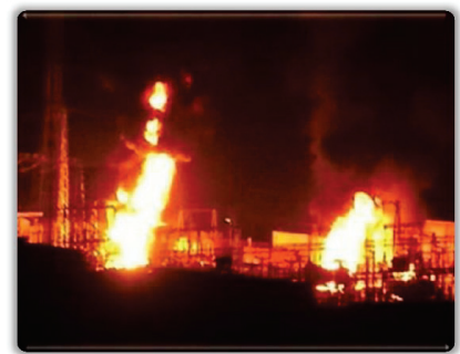
Fire caused by explosion of the MT
