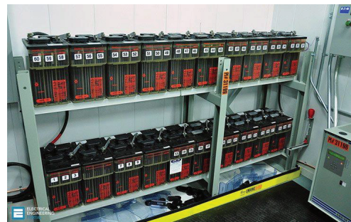
Photos from https://electrical-engineering-portal.com/substation-dc-auxiliary-supply-battery-and-charger-applications
