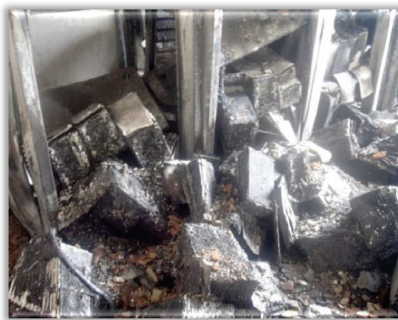
Explosion of batteries
