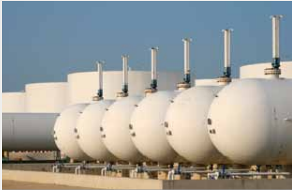
Petroleum storage tank standards are being updated as part of SCC's funding initiative.
